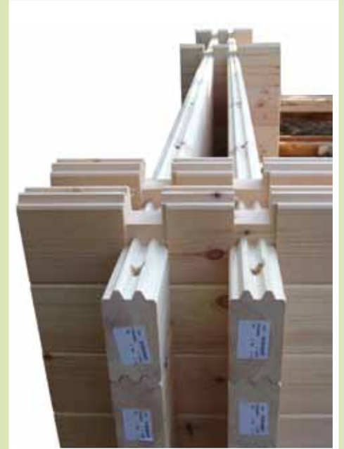
Twin wall structure - 2 x70mm logs.
